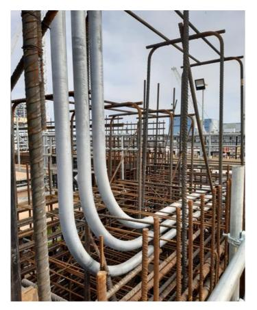
All embedded pipework and supports were installed and pressure tested by Ledwood.
